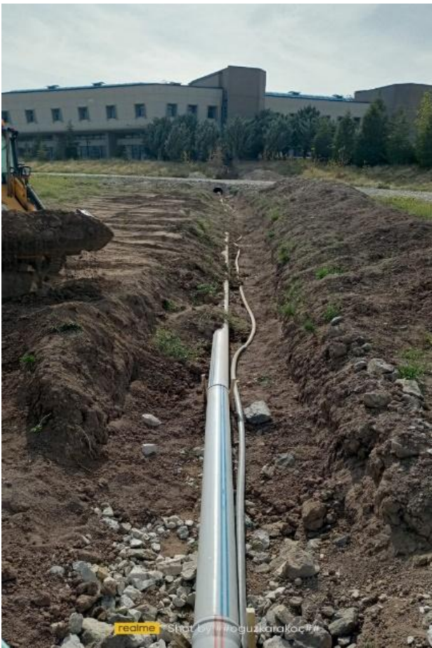
Figure 2 Images of the searched pipe and cable line before being buried
